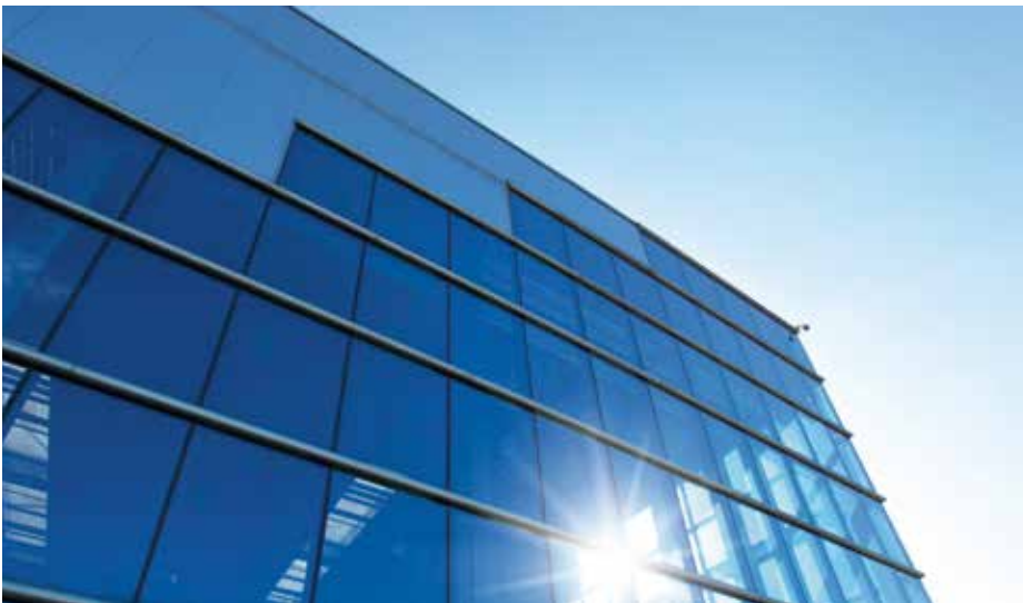
Modern office building with thin-film solar modules providing visual and heat protection
