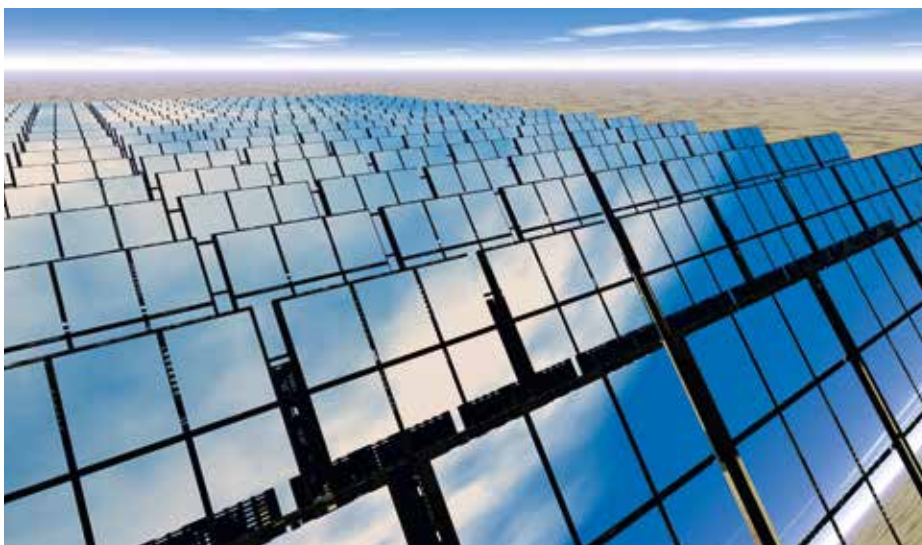
Large solar installation with thin-film solar modules
